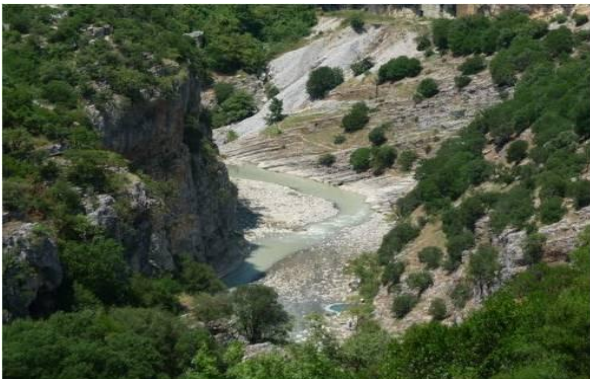
A Small Hydro Power Plant (SHPP) at Lengarica Canyon, managed by Enso hydro GmbH, an Austrian company, which received advisory services from IFC.
