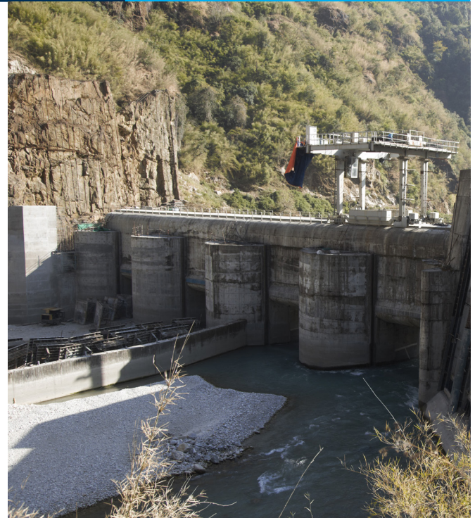
Construction underway at the 456MW Upper Tamakoshi hydropower project site, Dolakha.
