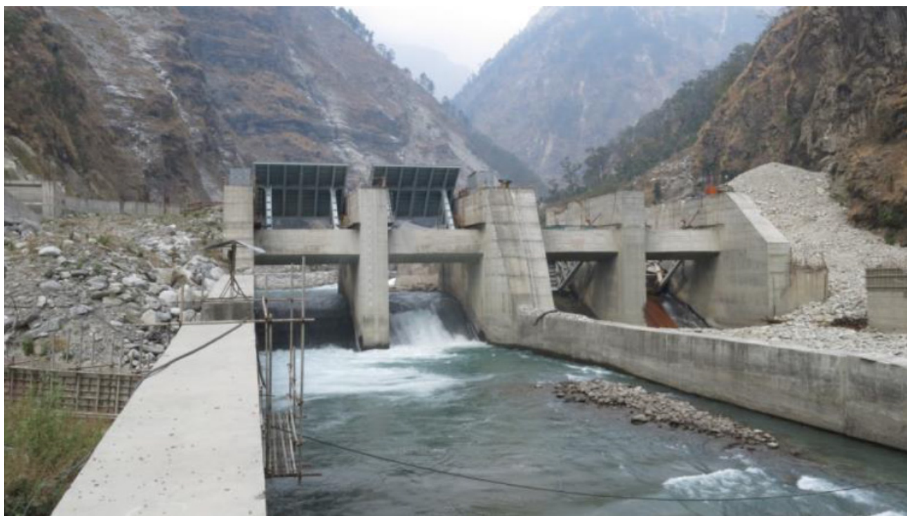
Photo D1.2: Dam Site of UT-3A, 2015
