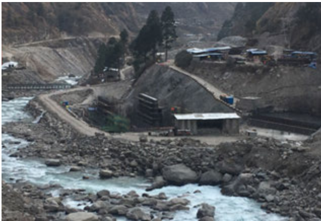
c. Construction activities for head works
