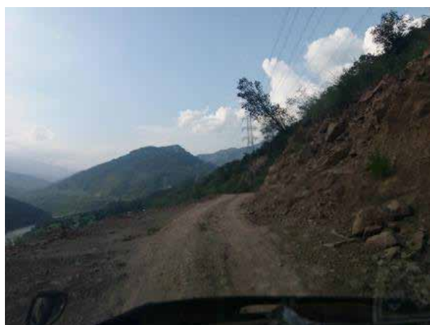
Sealed road covered with mud post landslide.
