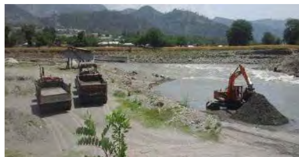
Sand mining with excavator
