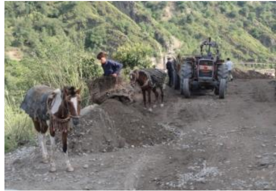
Sand Dumping on Road Side near confluence of Poonch River and Bann Nullah
