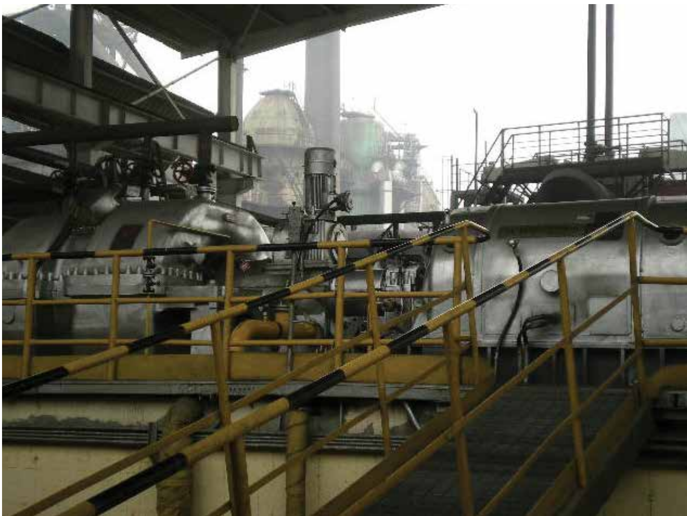
■ Sichuan Dazhou Steel Corporation installed new equipment that uses blast furnace gas to generate 28 gigawatts of power annually.
