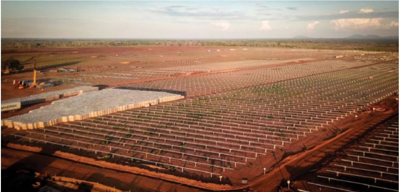
A 60 MW project being built in Malawi. The project creates 300 local jobs and is expected to contribute significantly with 20 percent of Malawi's current installed capacity.
