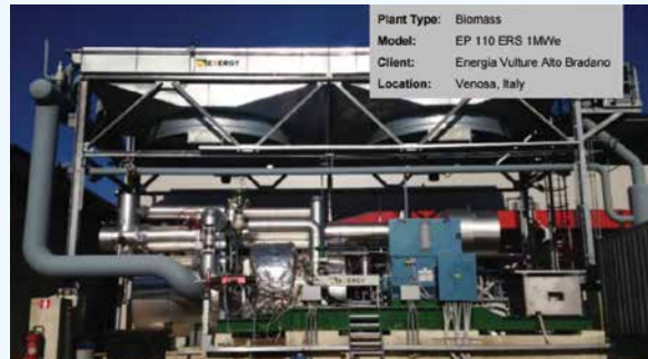
Figure 5-18: MWe Biomass-driven ORC Unit
