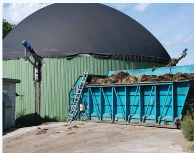
Figure 5-29: Biogas Plant with Integrated Gas Holding Tank Under a Soft Top
