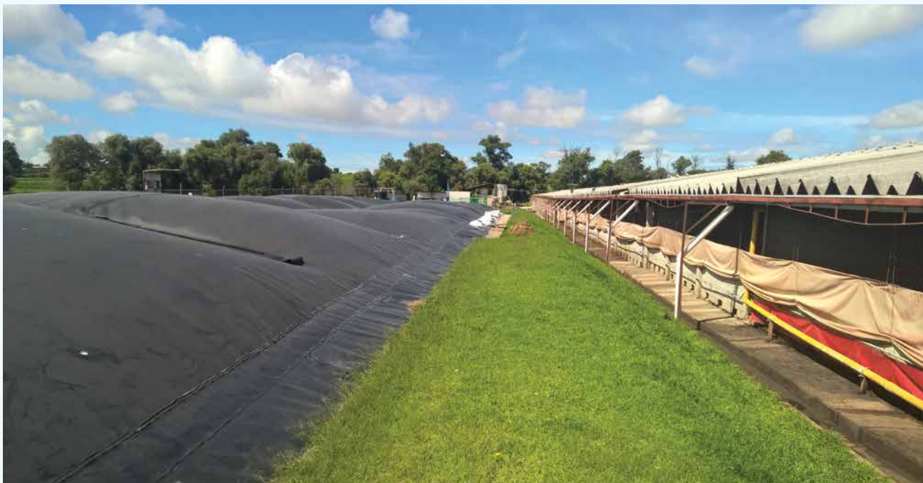
Figure 5-30: Biogas Production Based on Pig Manure and Slaughterhouse Residues Using a Lagoon Digester
