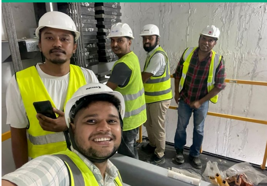
Workers at a Private Sector Window-supported data center in Nepal. Photo courtesy of WorldLink.
