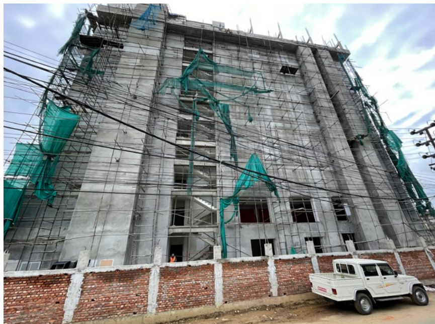
Construction is underway on WorldLink's data center in Nepal. Photo courtesy of WorldLink.
