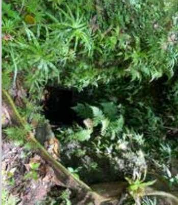
FORMER WWII BUNKER
