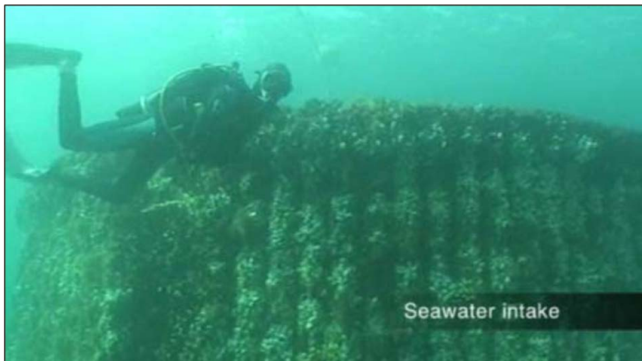
Figure 2-7: Macrofouling on screen of Intake Tower at Perth 1 SWRO plant
