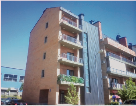
One of the resettlement buildings.
