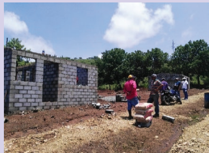
Building a new house in Nueva Jerusalén.
