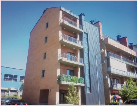
One of the resettlement buildings.
