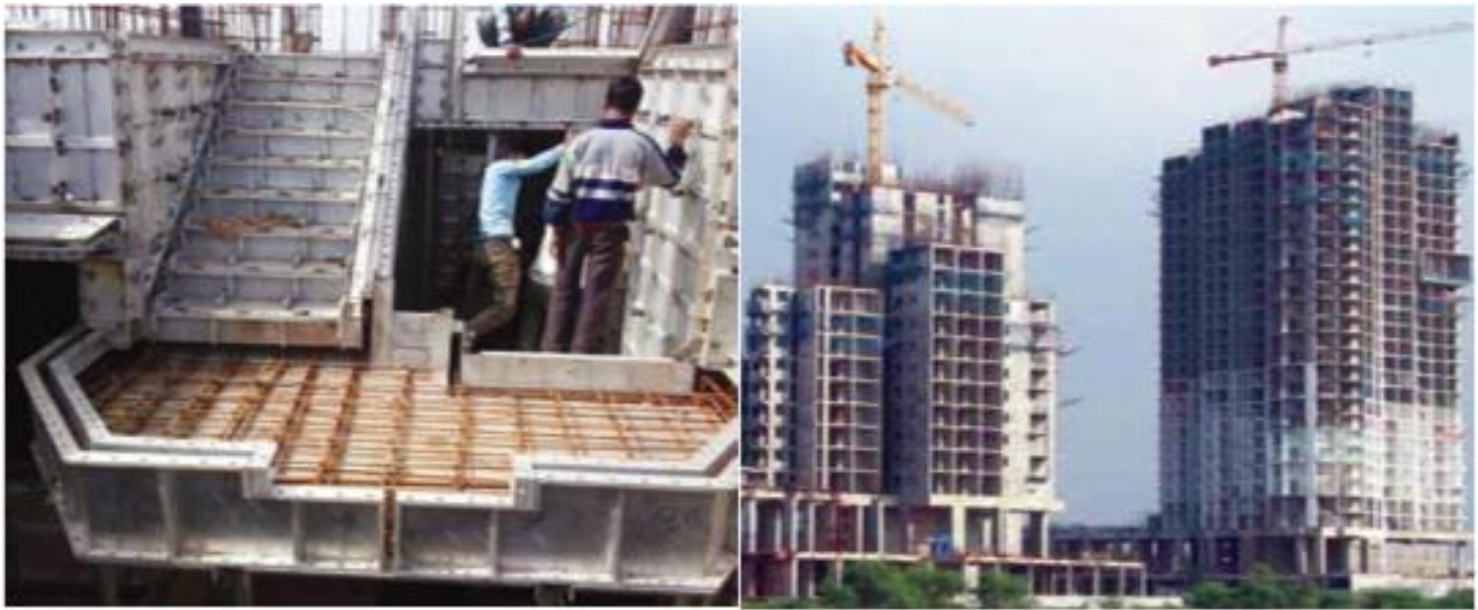
Figure 32: Monolithic concrete construction using aluminum formwork
