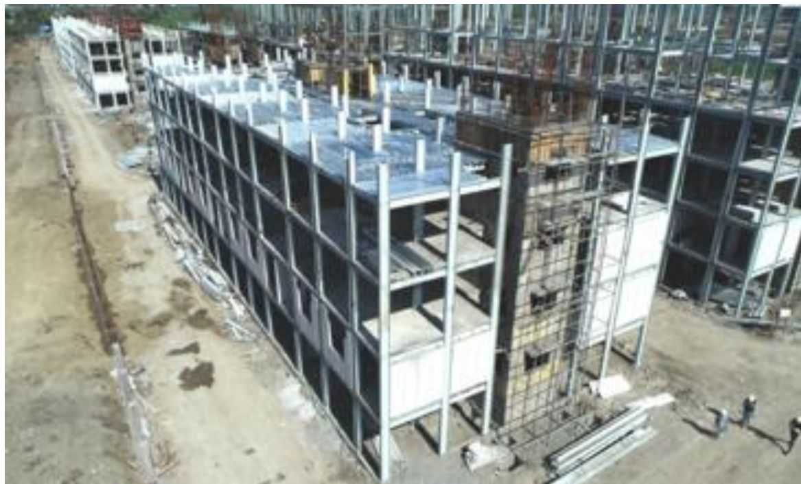
Figure 30: Progress of LHP in Indore using prefabricated sandwich panel system
