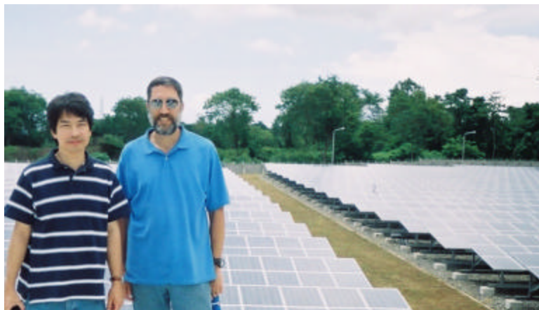
Stage 3: View of the Completed Facility – 1 MW of Capacity Alan Miller and the Project Manager in the foreground
