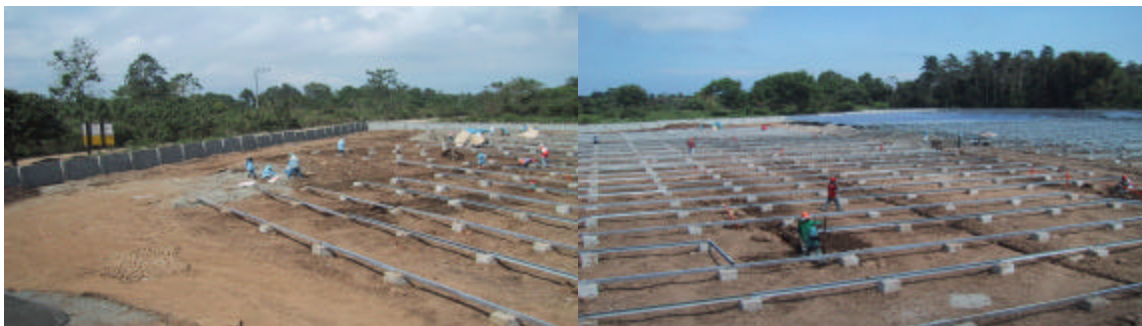
Stage 1: Initial Site Work
