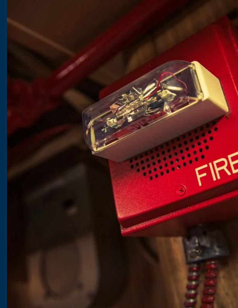
The maximum sound level in any location should not exceed 110 dBA. Visible notification means can be provided in areas with potential high noise levels (e.g., generator rooms).
