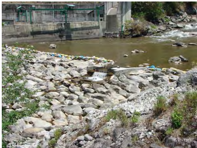
Khimti 1 Intake structure and low flow weir
