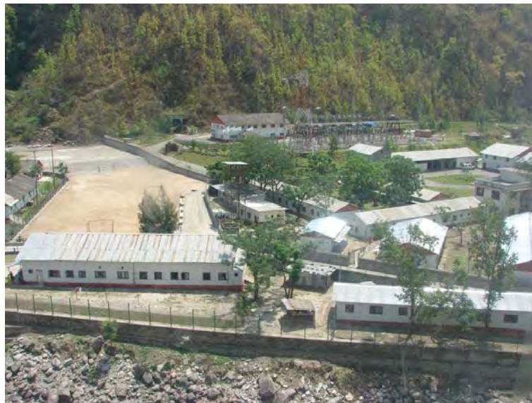
Khimti 1 Power House and Compound at Kirne
