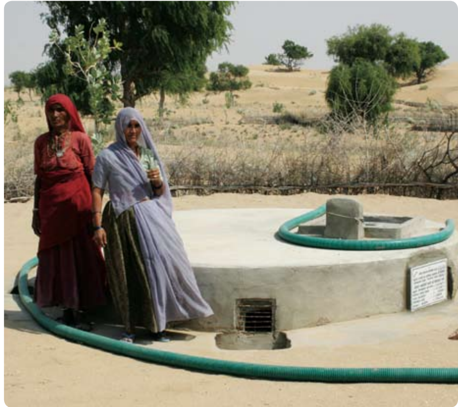
A rainwater collector well system developed as part of a technical assistance program in Rajasthan, India, will reduce the distance local women will have to walk for water.
