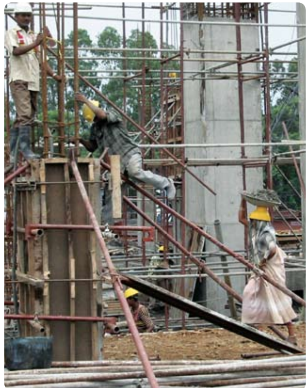
Work on the expansion of Andhra Pradesh Paper Mills in India.
